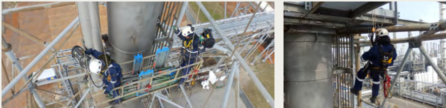
Utilizing rope access, suspended platforms and other alternatives to scaffolding enhances the safety of our people.
